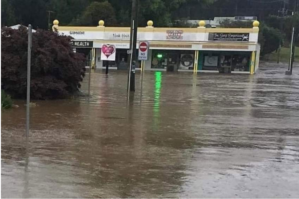
Image 4: The Princes Highway was flooded at Mogo, impacting shops on both sides of the road.
