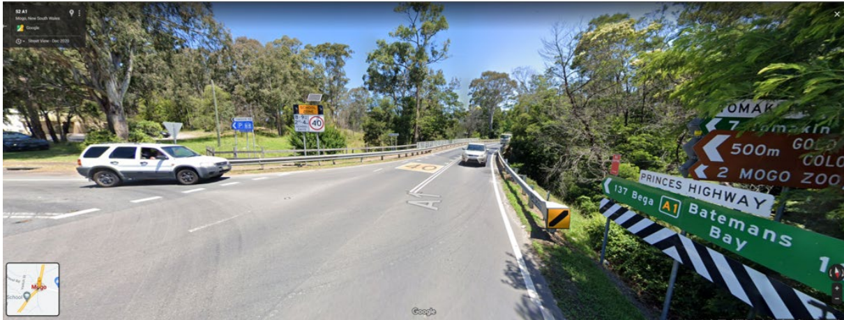
Image 11: Mogo Creek Bridge
