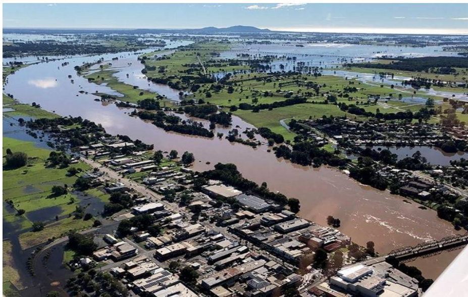
Figure 9: The Macleay River at the moderate level (around 5.7m) in Kempsey on the 24th March 2021
