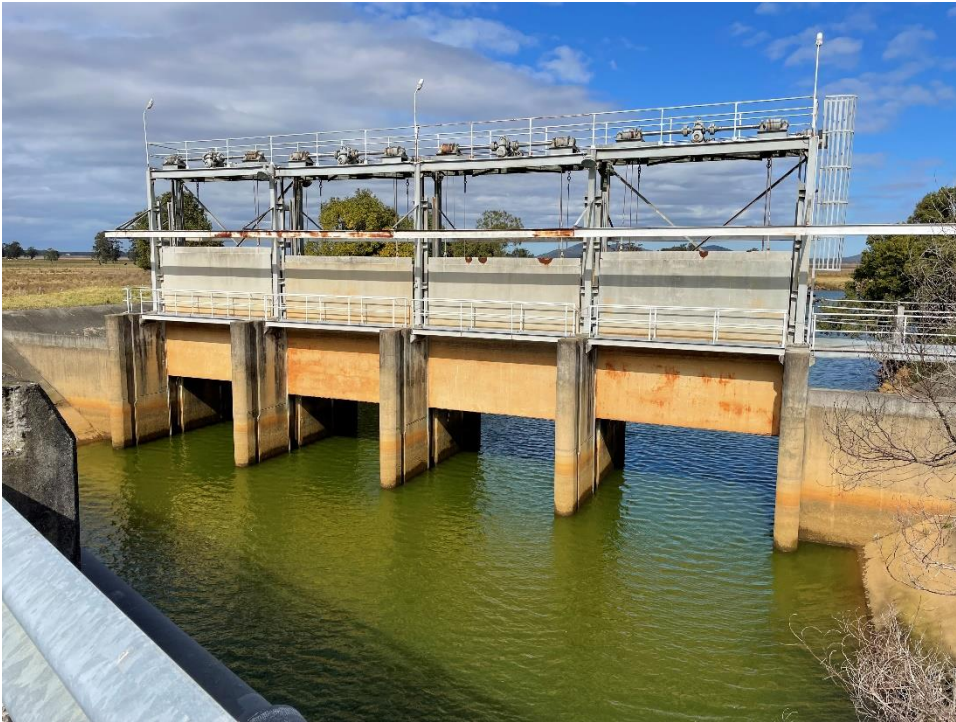
Figure 6: Belmore River and Kinchela Creek crossover gates
