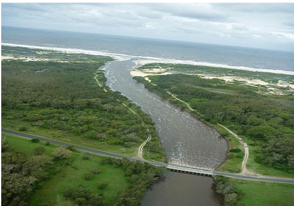
Figure 5: Ocean floodwater outlet discharging flood water from the Belmore area into the ocean.
